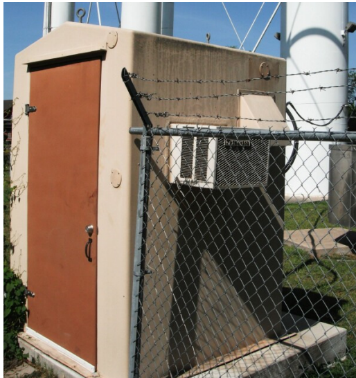
Melissa Repeater Hut
